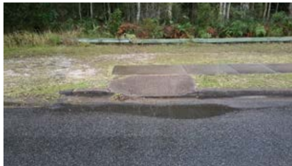
Visually DDA non-compliant kerb ramp: KR_00295
