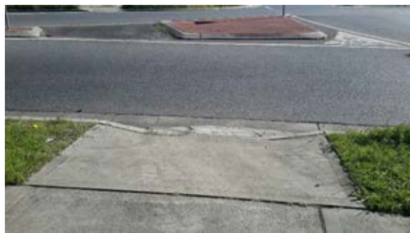
Visually DDA non-compliant kerb ramp: KR_00295
